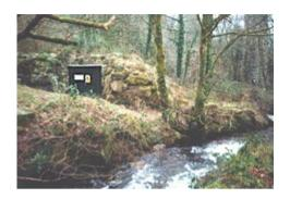
Hydro-electric powerhouse buried to reduce visual impact and noise
