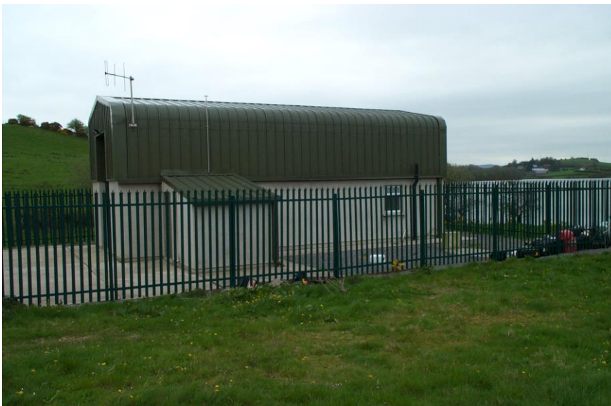
Fig. 1 - VWI's Dernakesh Water Treatment Plant.
